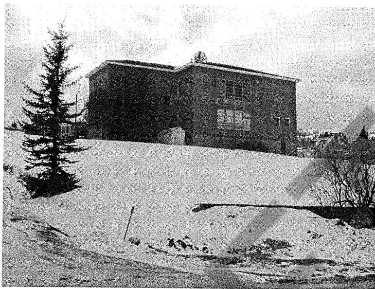
Looking southwest at the subject property from Wallace Street (Hwy 287) Photograph taken March 18, 2020 by J. Michael Joki, MAI, SRA
