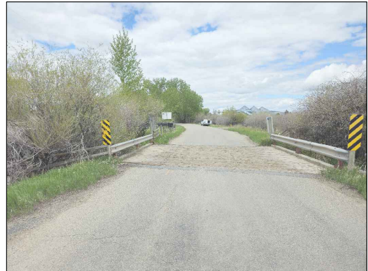
EXISTING BRIDGE APPROACH LOOKING WEST
